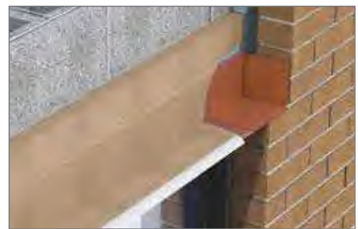
Thru-Wall shown with copper end dam (pg 42.)
